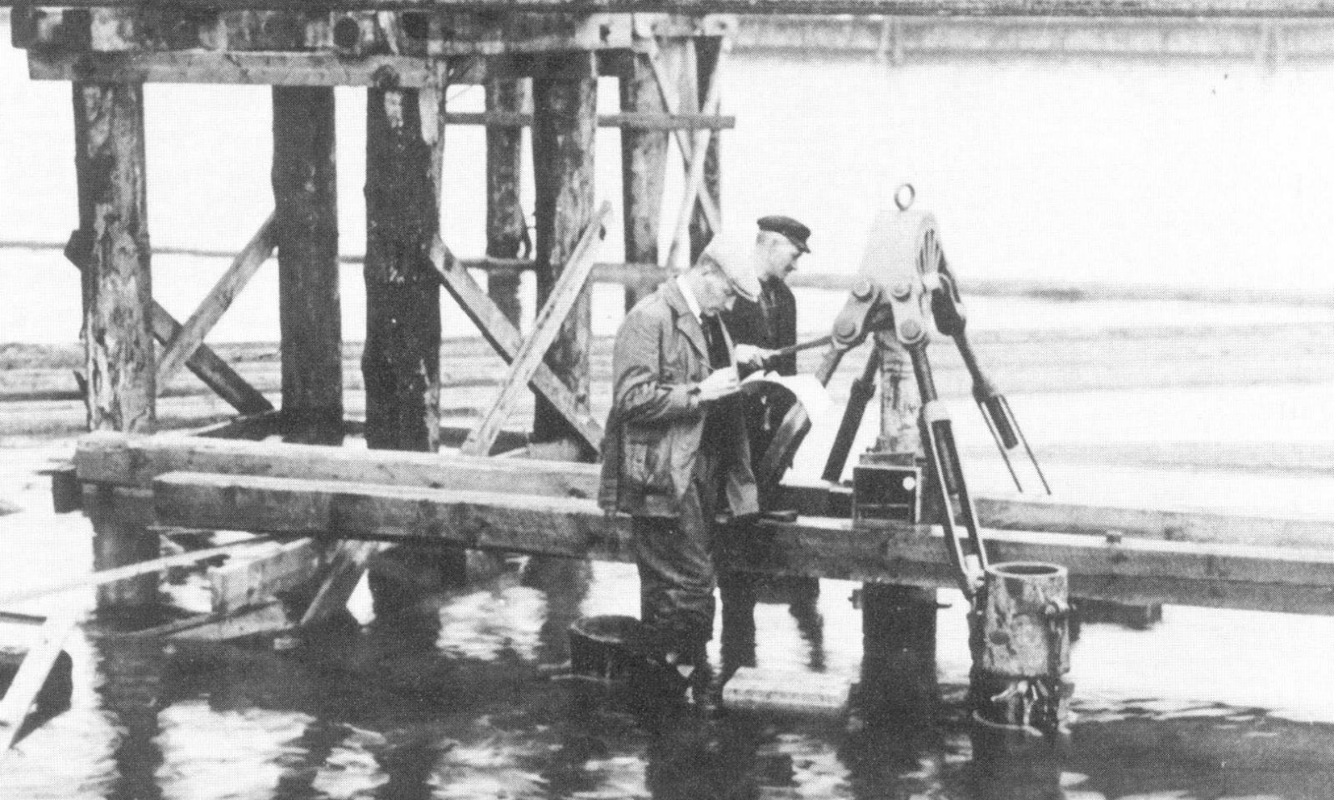
A static loading test performed in 1910 in Sweden by Mr. Wendel. Courtesy of Dr. Bengt Fellenius
